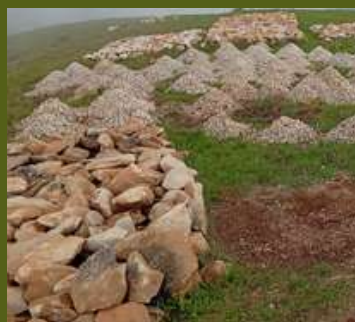
Pre-construction work at the Anape Field Station. Locally sourced rocks are chiseled to shape and size.
